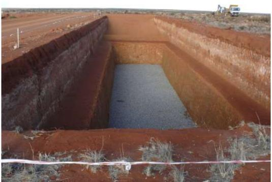
Figure 2: LLW near-surface disposal trench at Vaalputs
